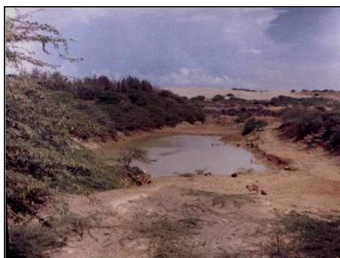
Fig. 2. Percolation Tank behind an earthen bund stores water in rainy season. The stored water recharges shallow aquifer for 3 to 4 months after the rainy season is over.
